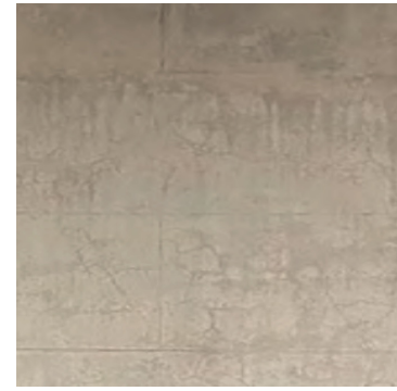
D Wall paint finish reference
