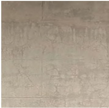
D Wall paint finish reference
